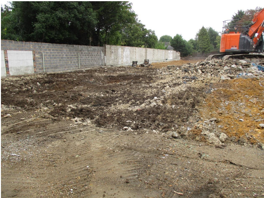
Plate 2 The northeast area of the site after the removal of the concrete hard standing
