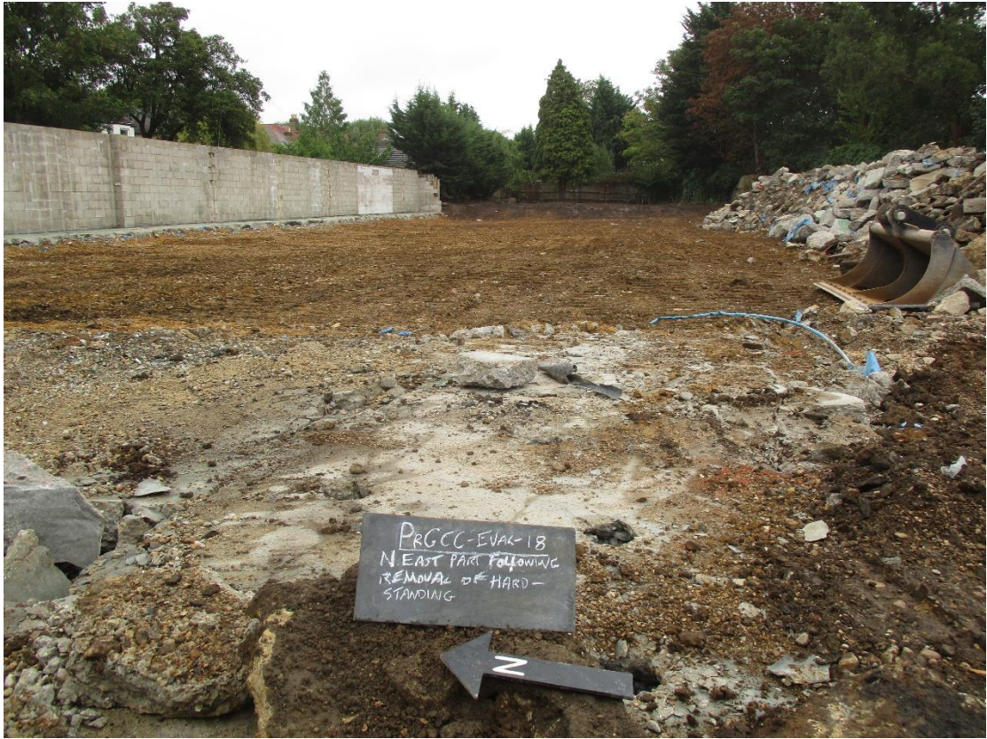
Plate 3 North-eastern are of the site following removal of hardstanding
