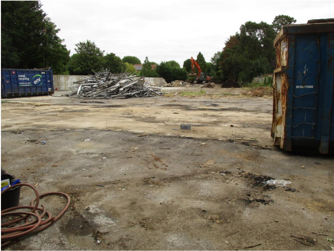
Plate 1 General view of Site, viewed from the east
